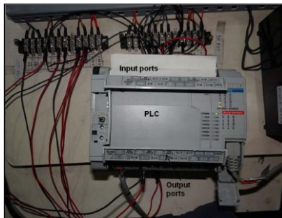
Basic Structure of PLC (Image)
